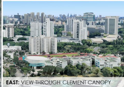
EAST: VIEW THROUGH CLEMENT CANOPY
